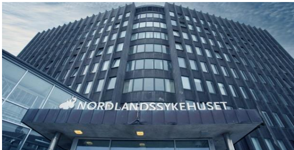
Nordland Hospital Bodø, Norway (2016)
